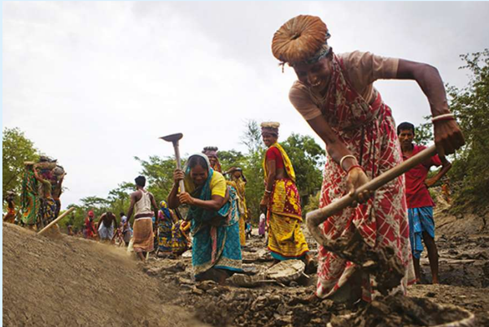
Labourers engaged in road construction
