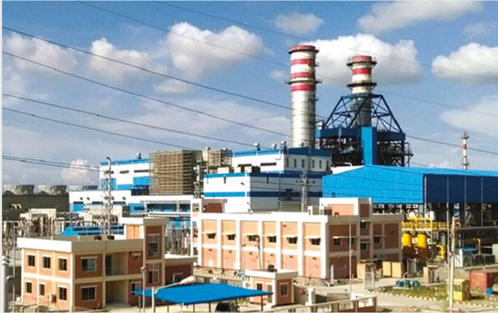
Bheramara 410 MW combined cycle power plant inaugurated on April 12
